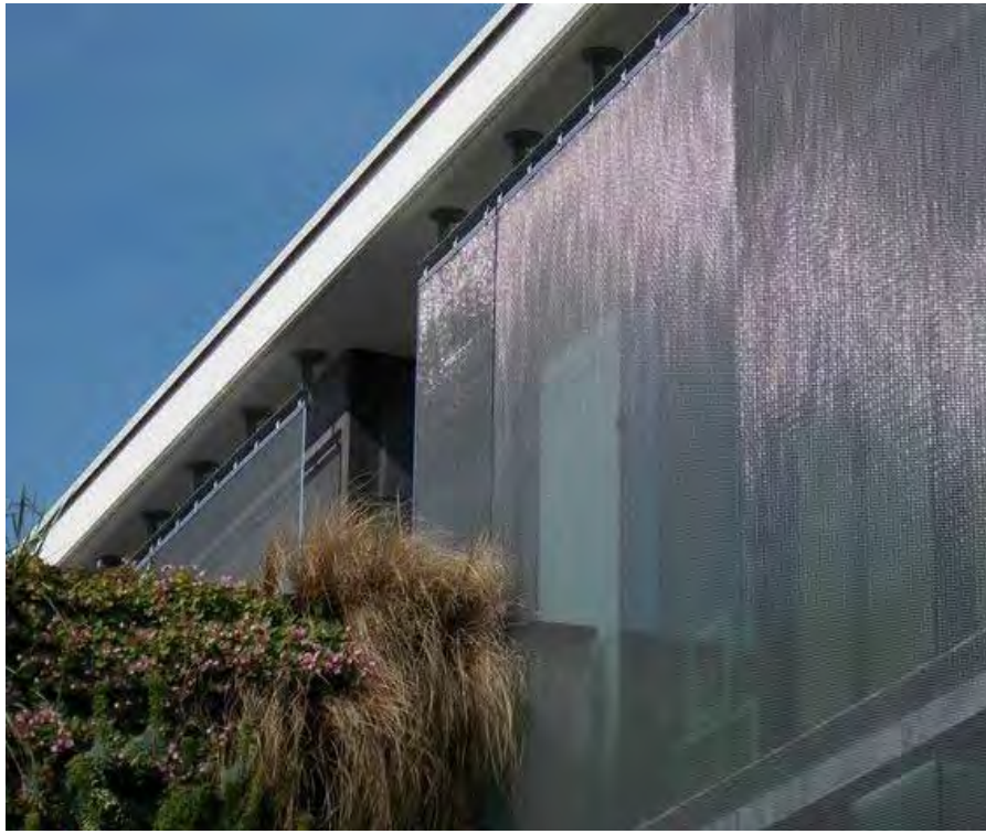
OPEN BATTENS AND MESH INFILLS
