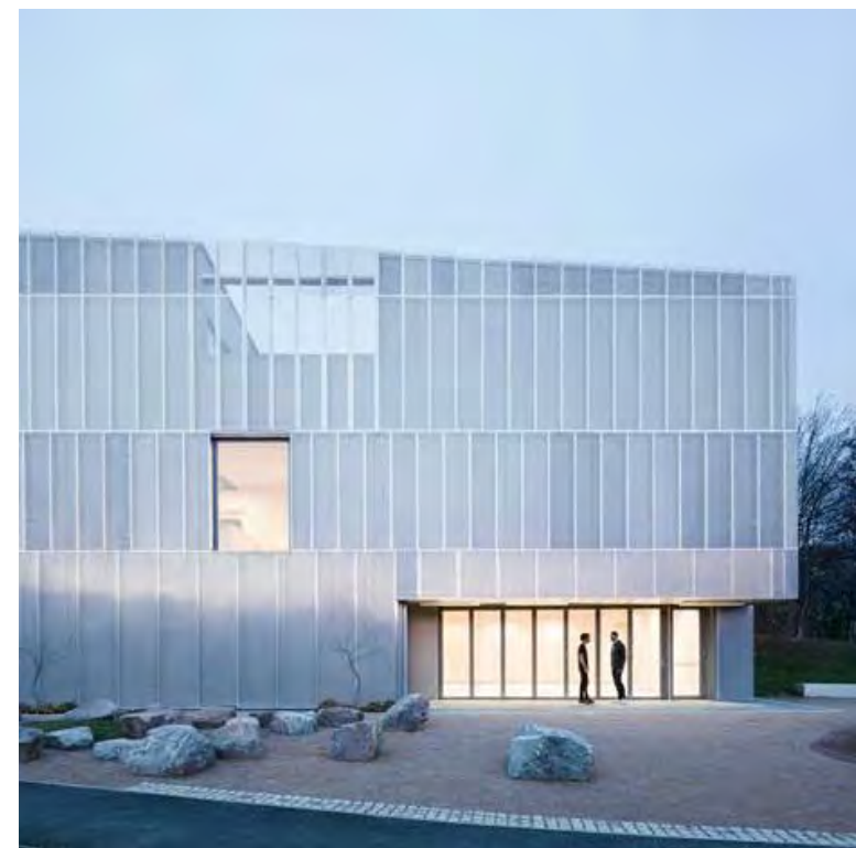
BATTENS WITH MESH INFILLS
